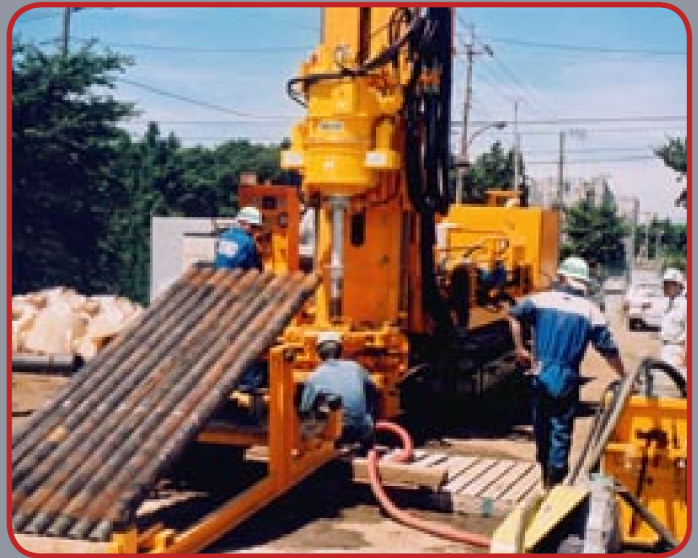
■ Injecting grout for soil stability improvement project.
