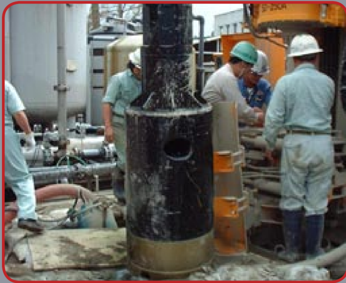
■ Drilling for the installation of a large diameter dewatering well.
