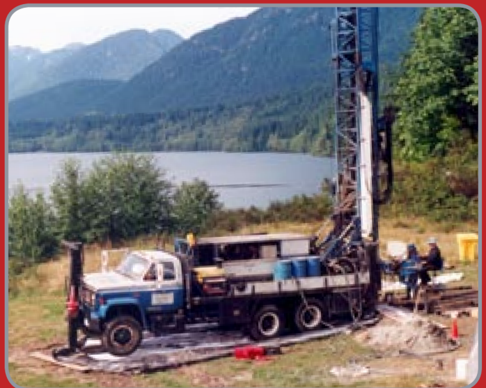
■ Installing piezometers to monitor seepage from a drinking water reservoir.
