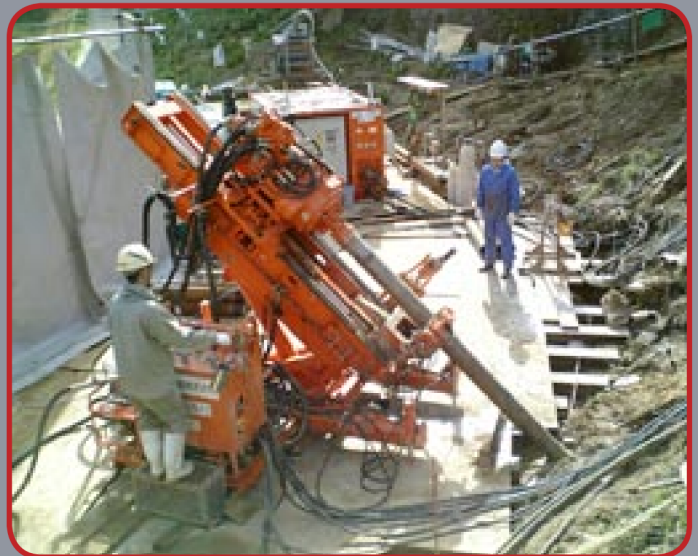
■ Installing anchors for landslide prevention.
