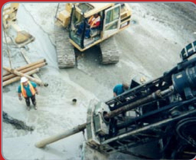
■ Injecting grout in old mine workings to prevent subsidence of above ground structures.
