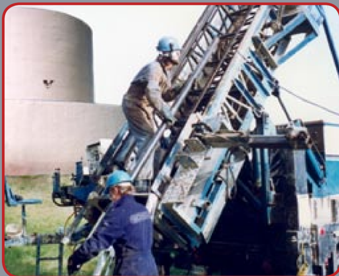
■ Angle drilling for the installation of cathodic protection anodes under a liquid natural gas steel storage tank.
