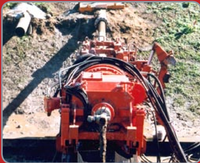
■ Horizontal continuous core drilling, with reverse circulation, for tunnel pre-boring assessment.
